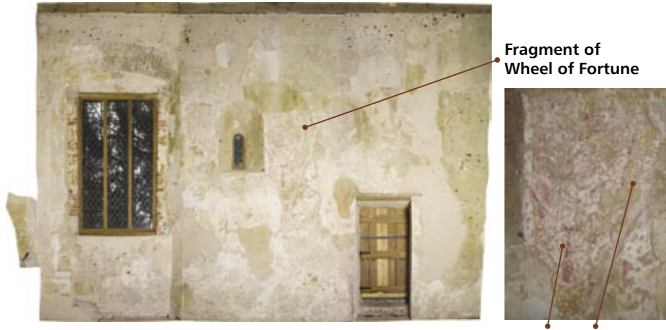
Fig 21: South wall: Wheel of Fortune
