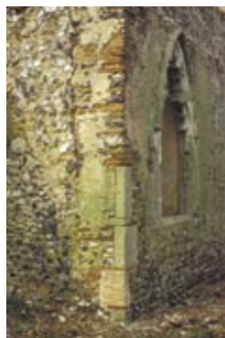
Fig 10: Long and short work and Roman brick, 'a' on plan
