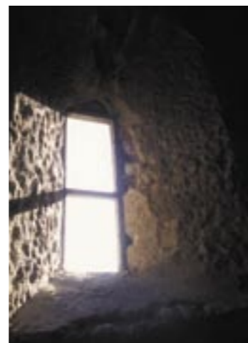
Fig 11: Double-splayed window, 'b' on plan
